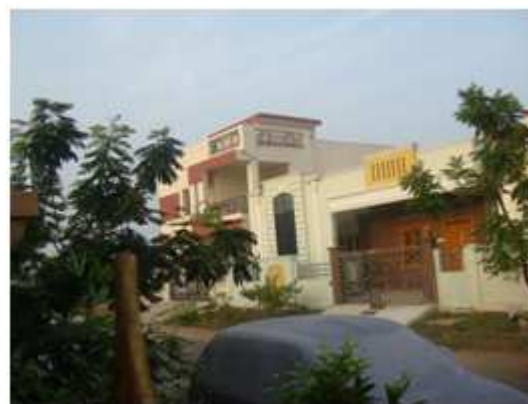
Figure 2: The Picture Giving the Information about the Road Shoulder Beside to the Bitumen Road in the Colony. Photo by Author
